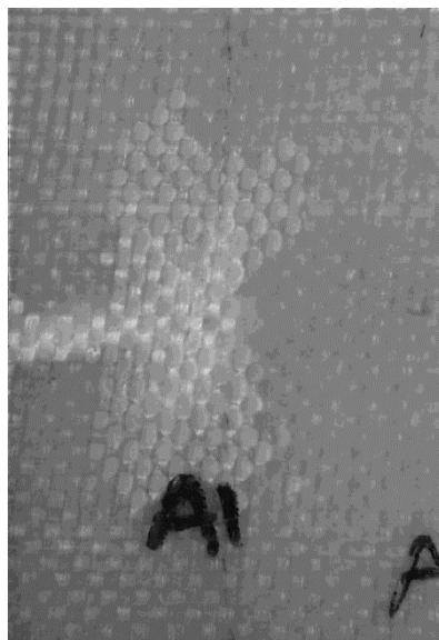
Fig. 4. Front face code 2: butterfly delamination with shear cracks.
