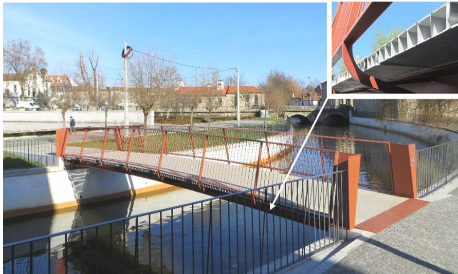
Fig. 1. S. Mateus GFRP-steel hybrid footbridge, Viseu, Portugal [1].
